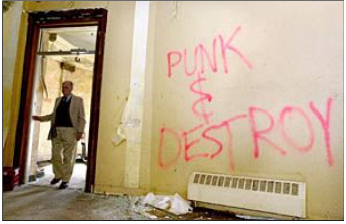
Bernie Levy of Binghamton takes a look around the Kilmer Building at Lewis and Chenango streets. Rep. Maurice Hinchey announced plans Wednesday to convert the Binghamton building into apartments and commercial space.
